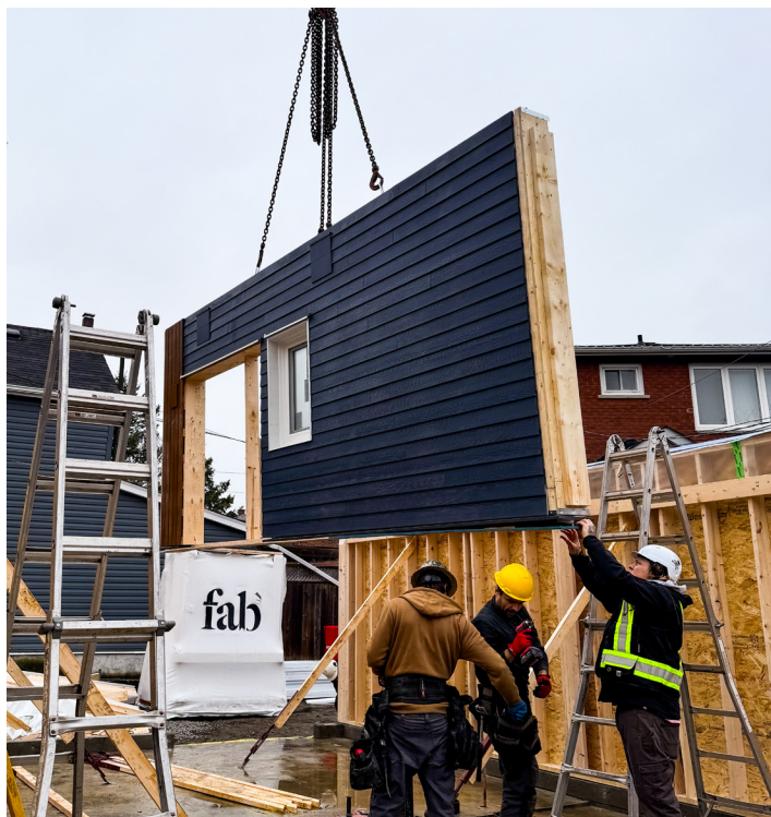
Fig 3. A factory built prefabricated wall component being assembled at a construction site in Toronto. Source: Assembly Corp.
