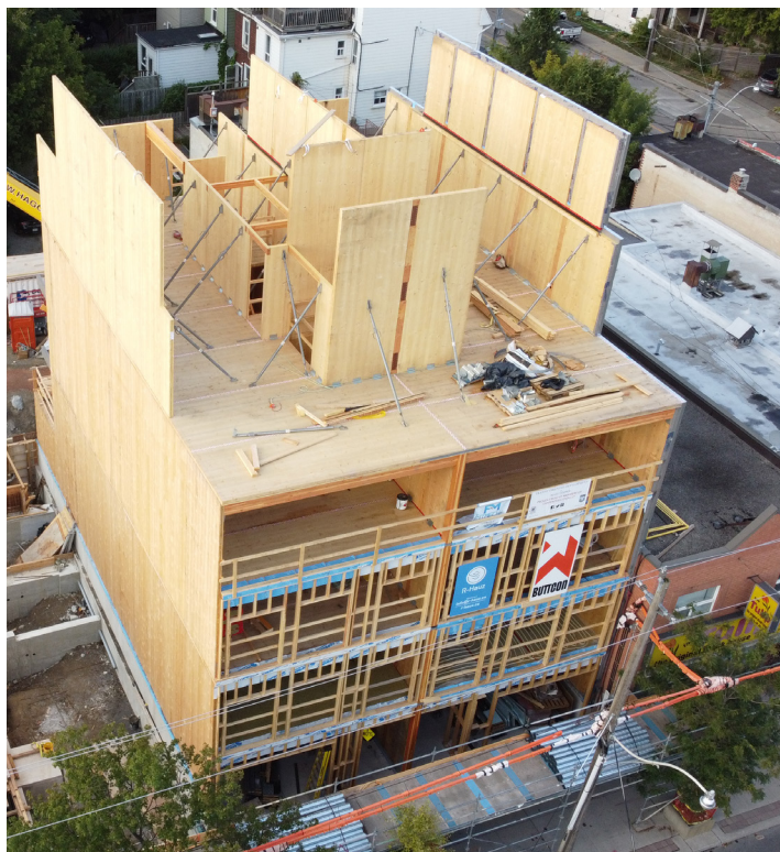
Fig 6. Factory built components being installed at a construction site in Toronto; Source: Assembly Corp.
