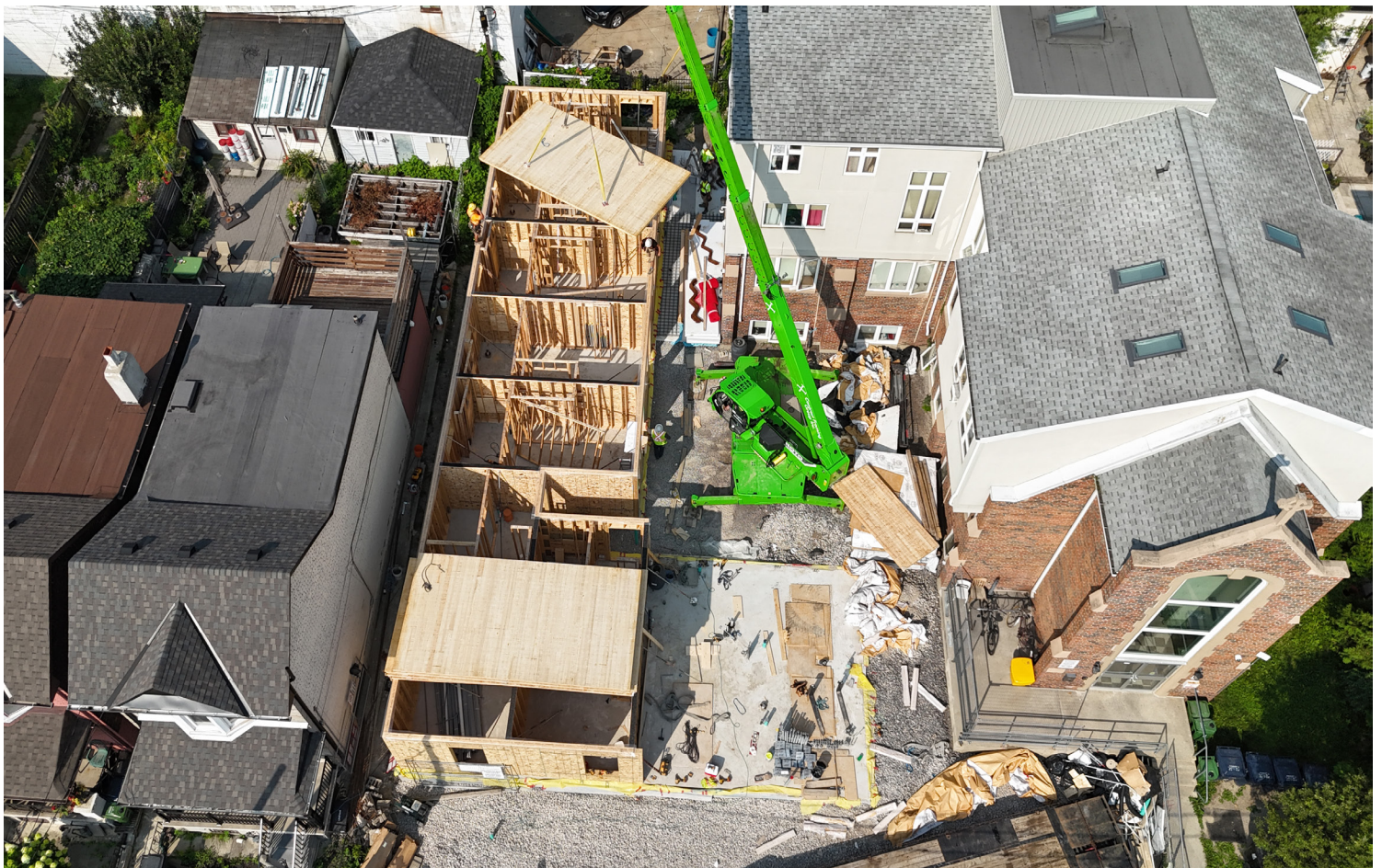
Fig 2. An infill development project in Ossington, Toronto uses prefabricated modular construction. Source: Assembly Corp.
